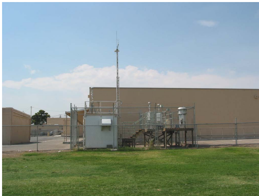
Figure 53. J.D. Smith Monitoring Station.
