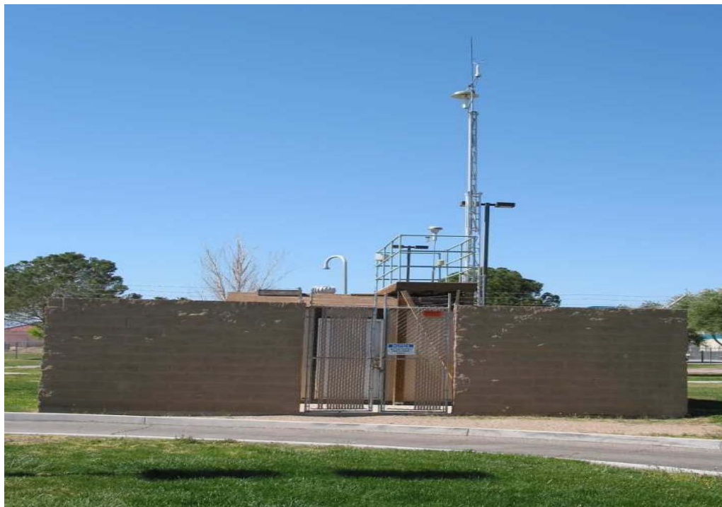
Figure 43. Paul Meyer Monitoring Station.
